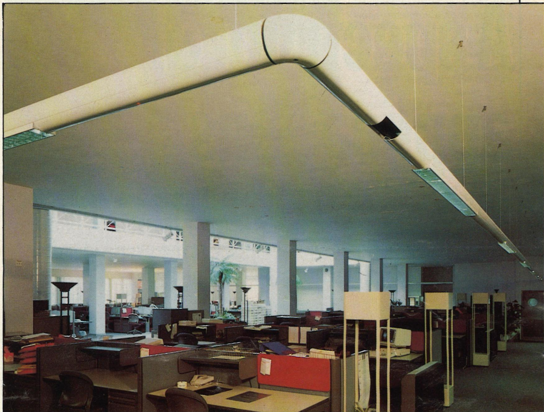
A view of one of Freemans' offices showing the BIS linear lighting system.
