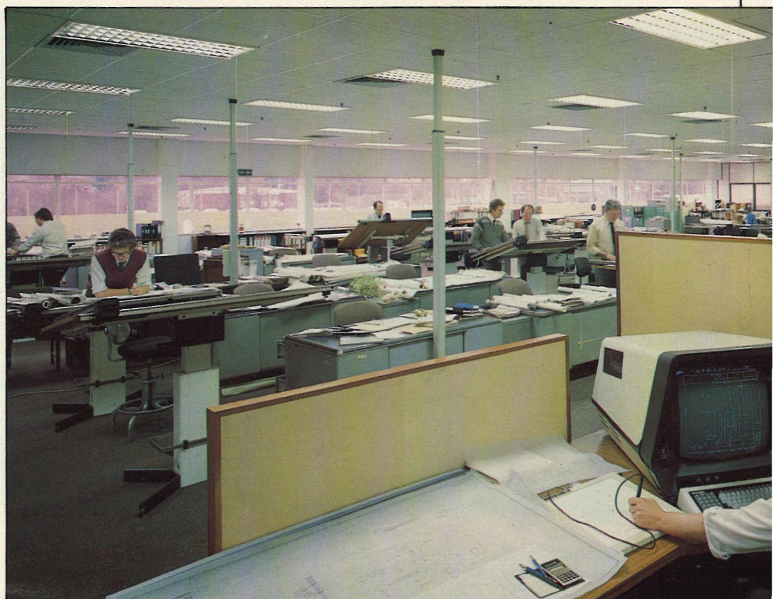
Recessed fluorescent fittings with low brightness louvers light the drawing office at Lucas Girling Ltd.
